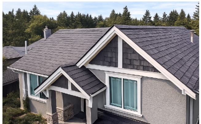
Left front roof slope and entry overhang
