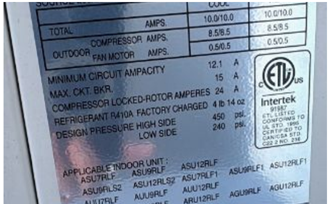
Manufacturer data plate for outdoor unit
