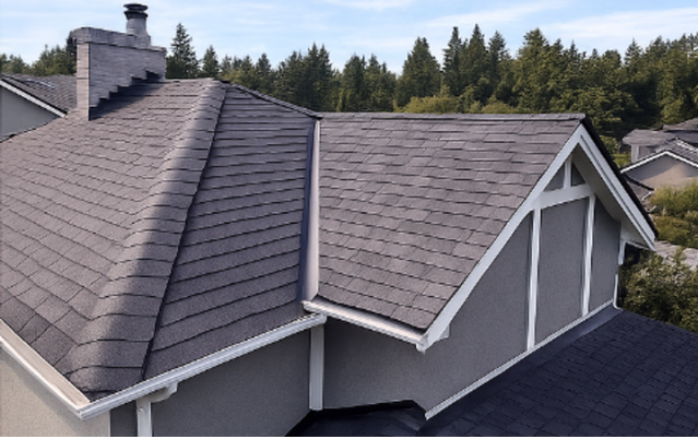
Rear roof slopes, ridge line, and intersecting gables
