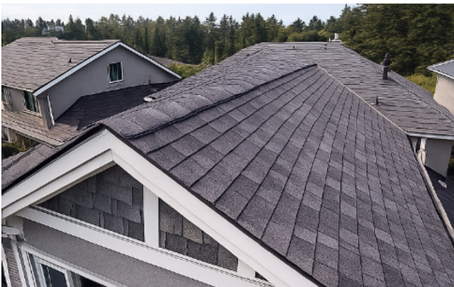
Main upper roof slope and valley intersection
