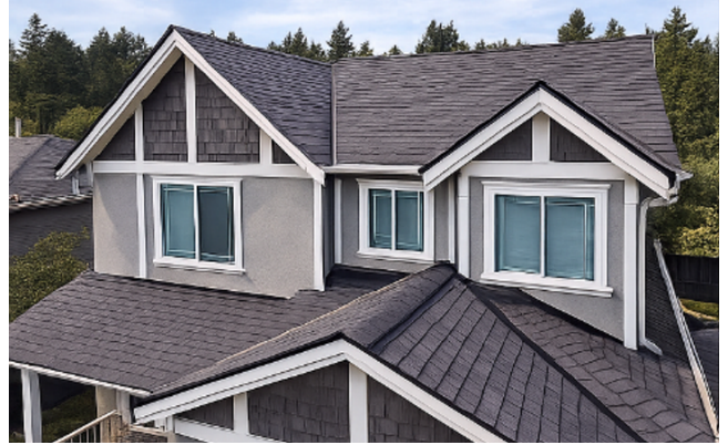
Front-facing roof slopes and gables
